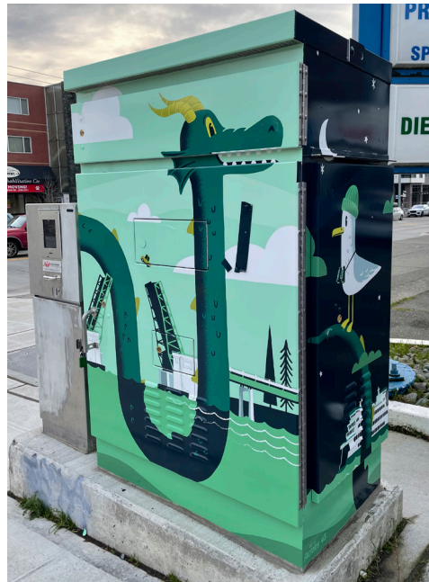
COMPLETED UTILITY BOX ON NW CORNER OF NW MARKET ST & 24TH AVE
